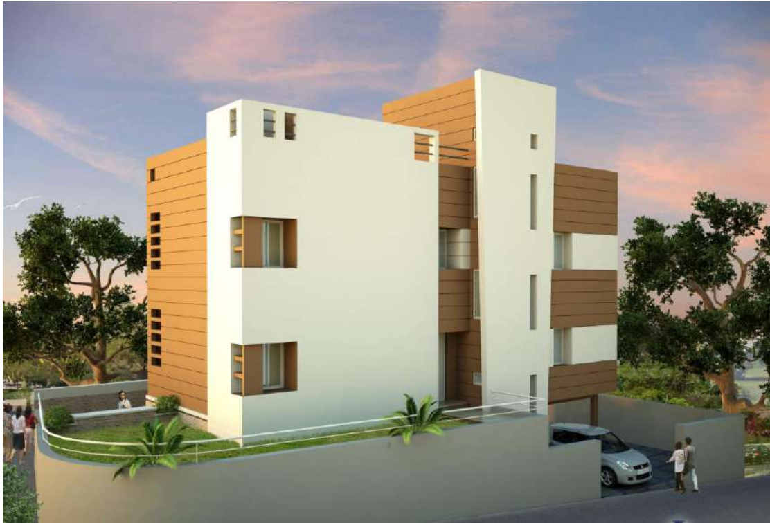
For Client B. K. Deshpande, Panchgaon road, Kolhapur
